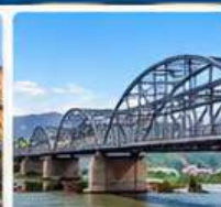
YELLOW RIVER IRON BRIDGE
